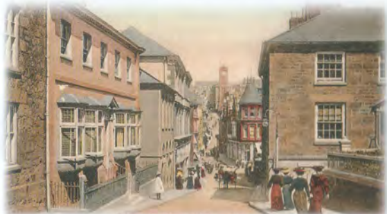
West End and Fore Street
